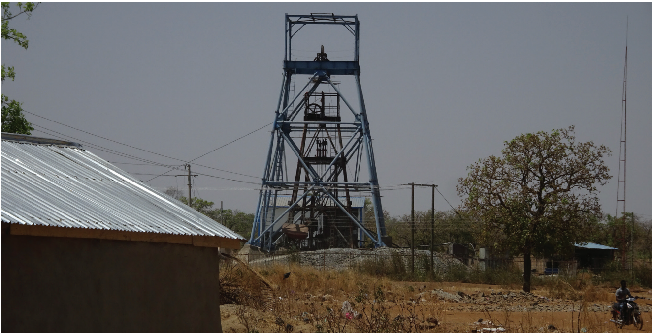
Figure 20 Headgear above shaft of the Chinese mining operation. Kejetia, January 2020.
