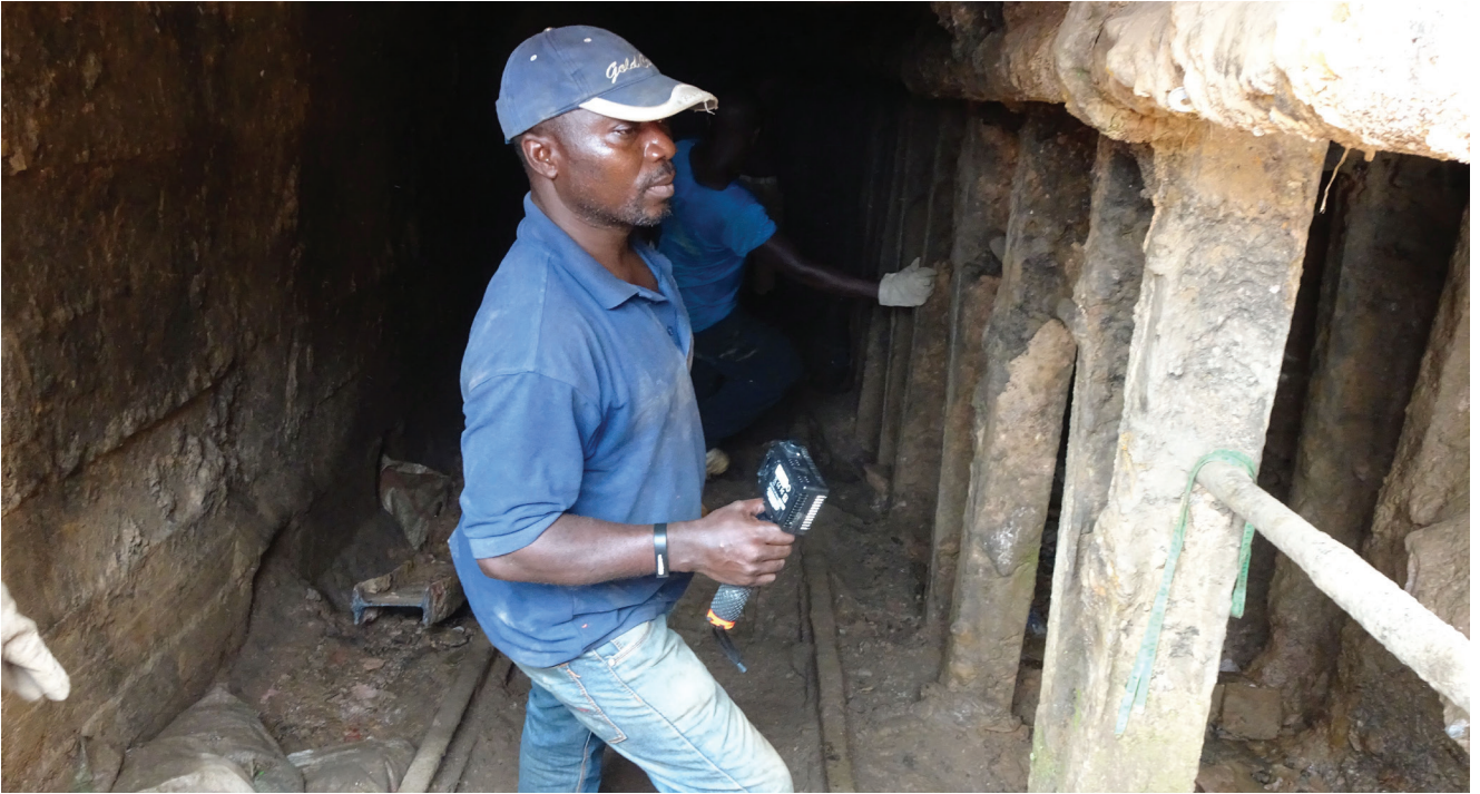
Figure 11 Filming renewing old infrastructure. Tarkwa, March 2018.
