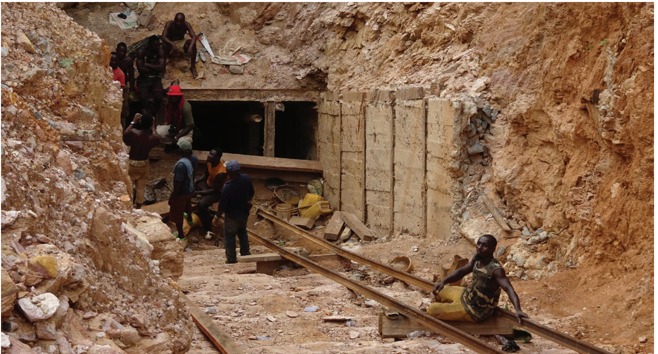
Figure 10 Renewing old infrastructure. Tarkwa, March 2018.
